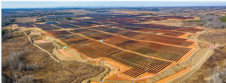
Solar facility under construction in Spotsylvania County. Photo Credit: Hugh Kenney, Piedmont Environmental Council
