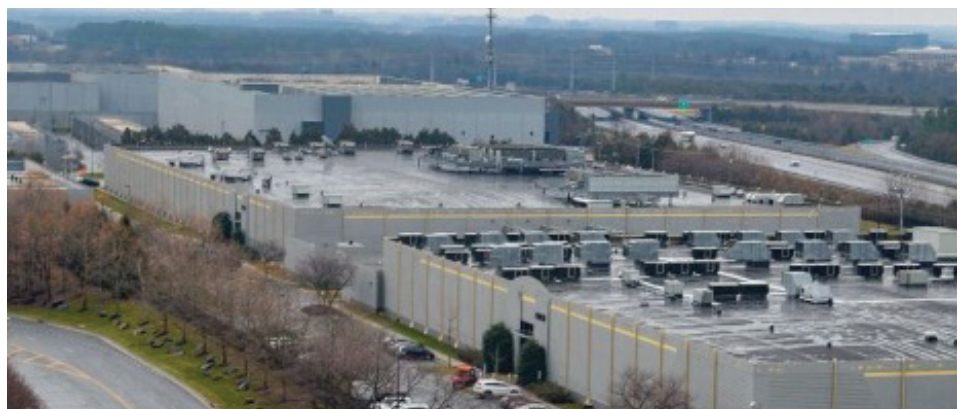
Data Center Alley - Loudoun County
