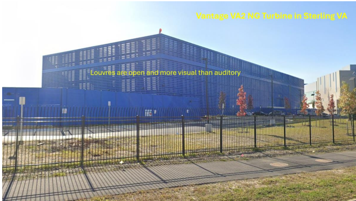
Figure 4. The Vantage roofless turbine building covers 1.5 acres and is about 50 feet tall. The noise emissions have been described by local residents as a continuous whine, with decibel readings exceeding Loudoun County's thresholds.
