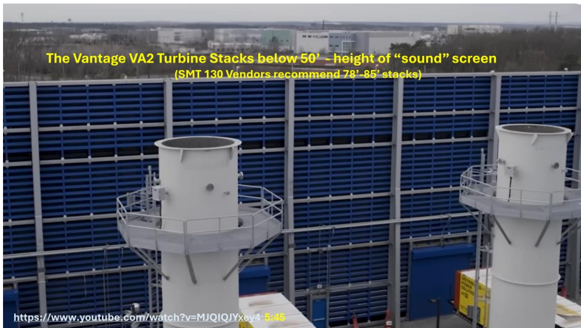
Figure 3. 50' Louvered surrounds are used to reduce visual impact with little impact on
