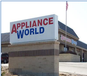
Not Allowed: Base and sign are not proportionate and there is no landscaping present.
