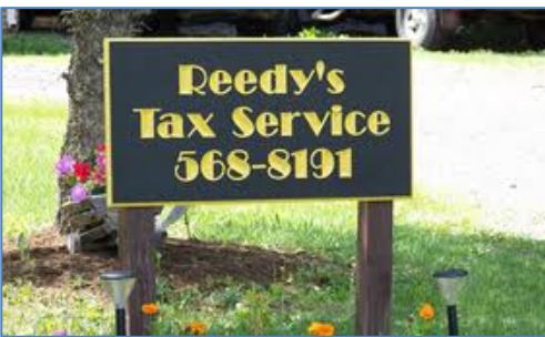
Not Allowed: Sign face is not attached on the inside of the supporting structure.
